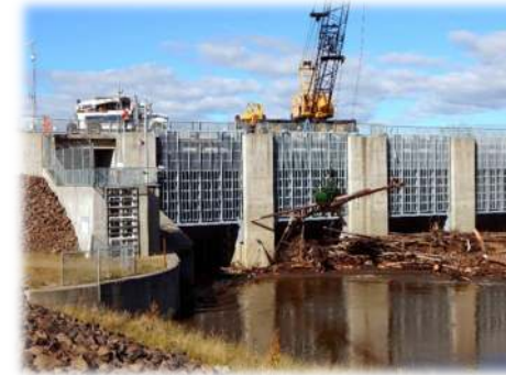
Moose Creek Dam Modification IIJA $88.5M Total Cost: $153M, Awarded 2021
